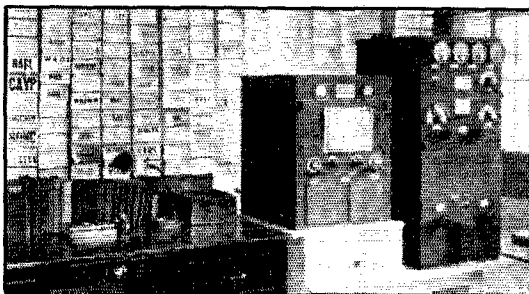
THE TRANSMITTER AT W5OW-WLJ
